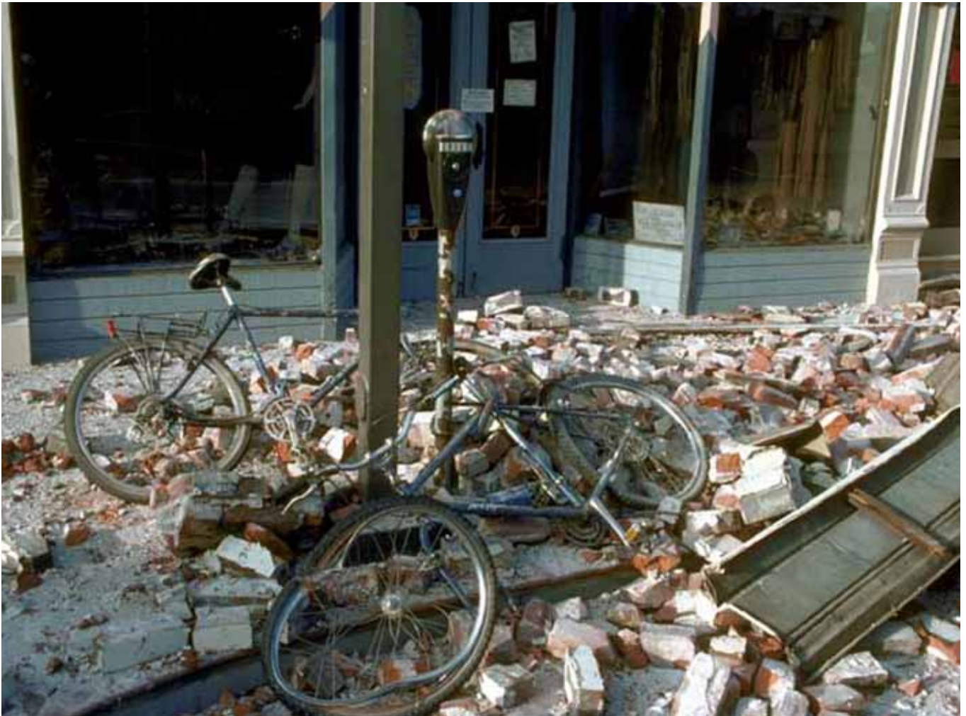
■ 1989 LOMA PRIETA EARTHQUAKE: Bicycles are crushed by falling unreinforced brick facade, Santa Cruz, Calif.
